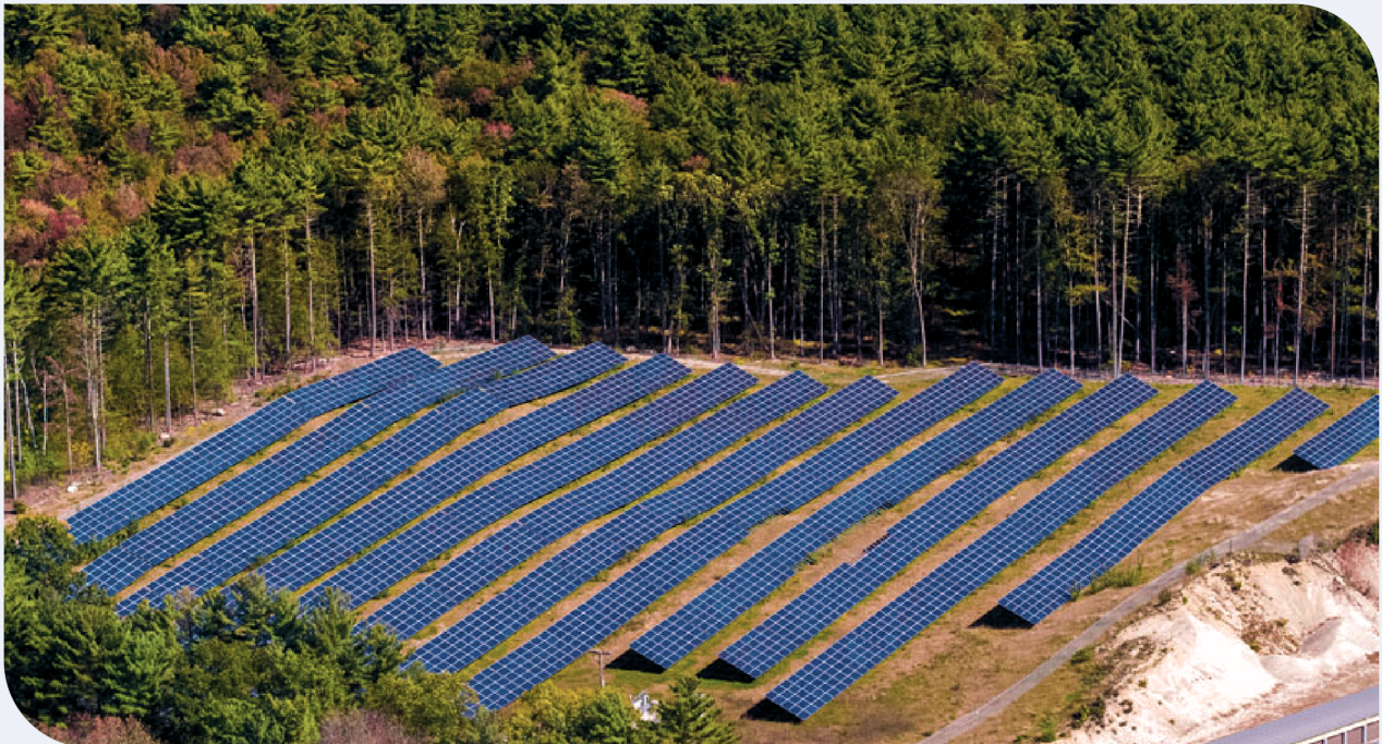
COMMUNITY SOLAR FARM PROJECT MASSACHUSETTS
